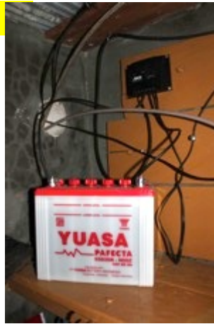
Batteries and charge controllers
