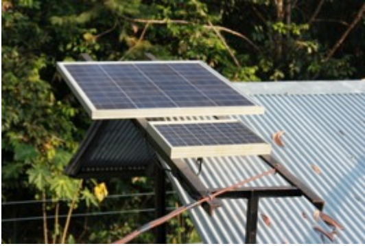
Solar panels to charge batteries
