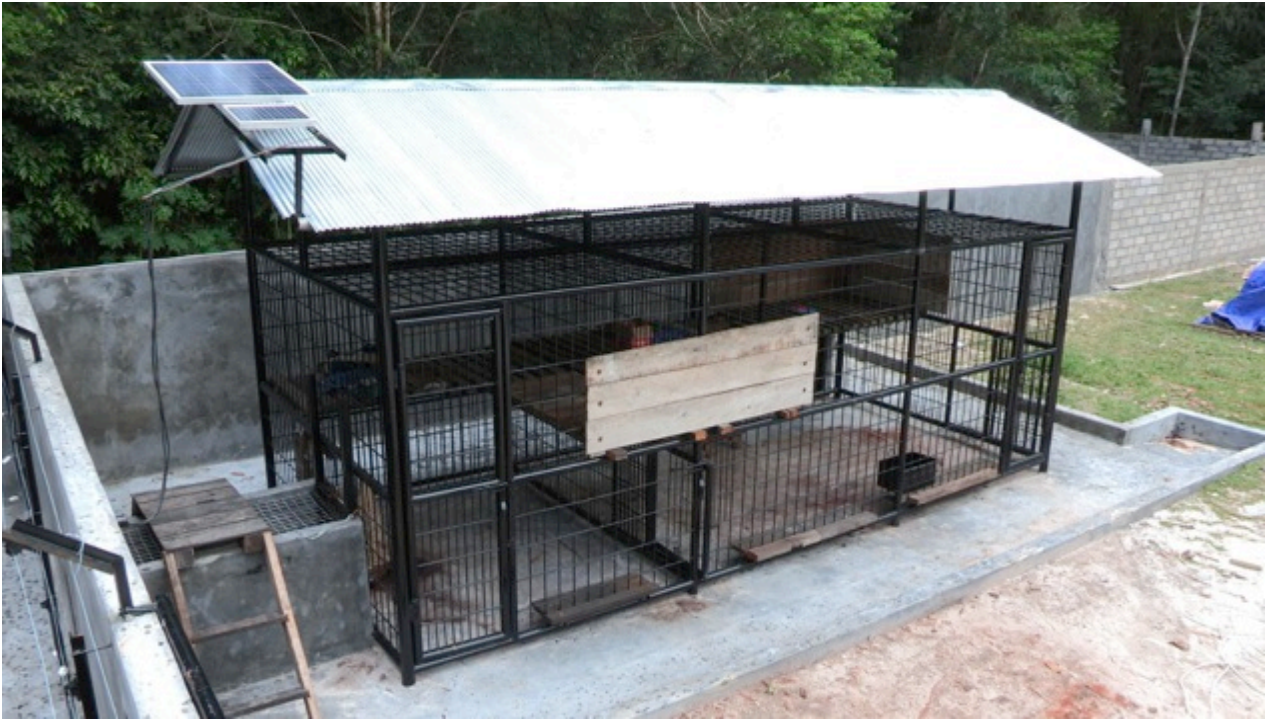
Feeding cage with 2 compartments for a total size of 2,5 m x 6 m and a height of 2 m.
